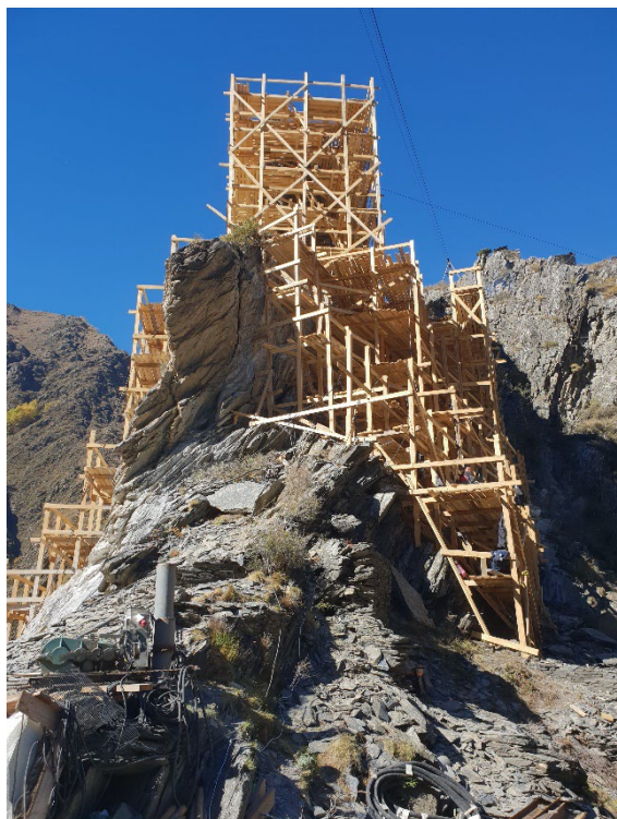
Figure 4. Photo taken in 2018 during restoration
