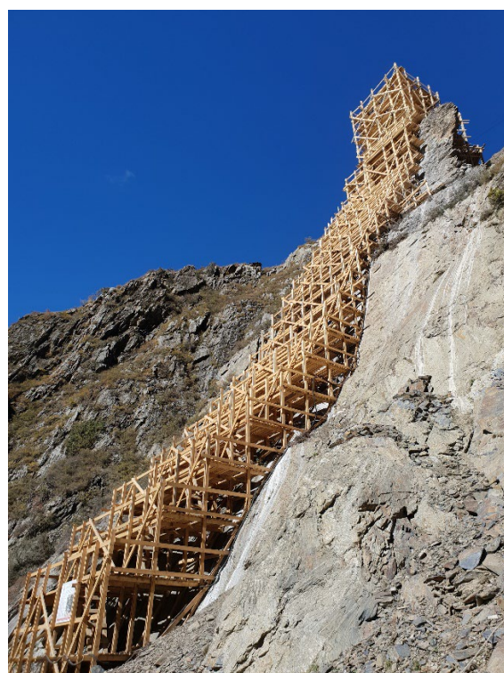
Figure 5. Photo taken in 2018 during restoration
