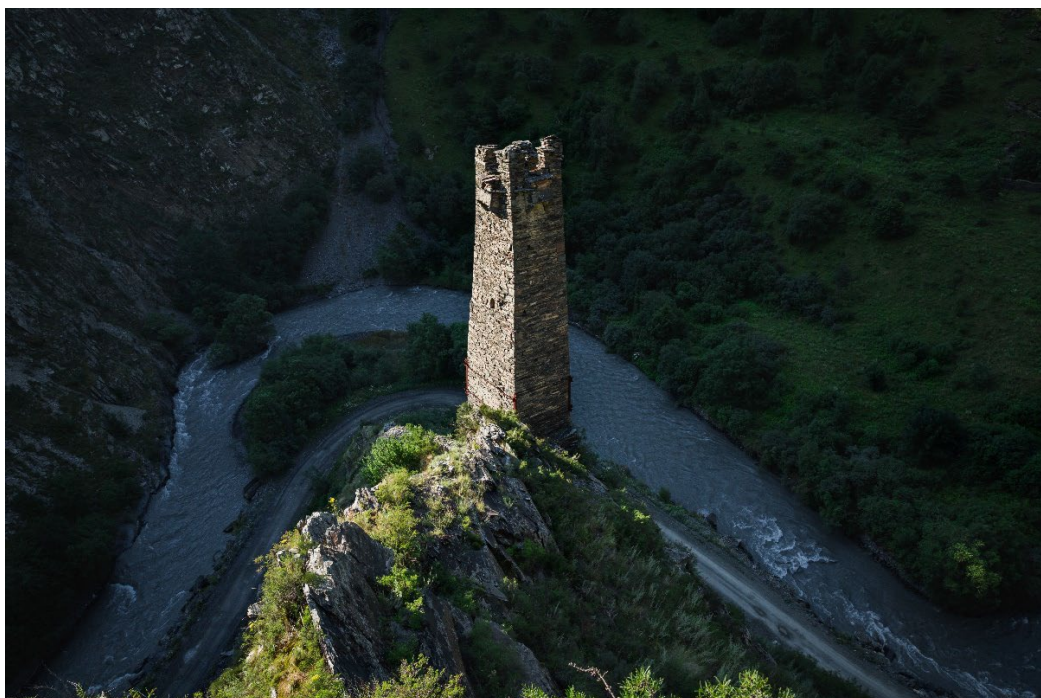
Figure 2. Photo taken in 2017 before repair and restoration
