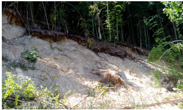
Figure 02. Head scarp of the landslide (photo by C.-D. Ursu, 2019)]
