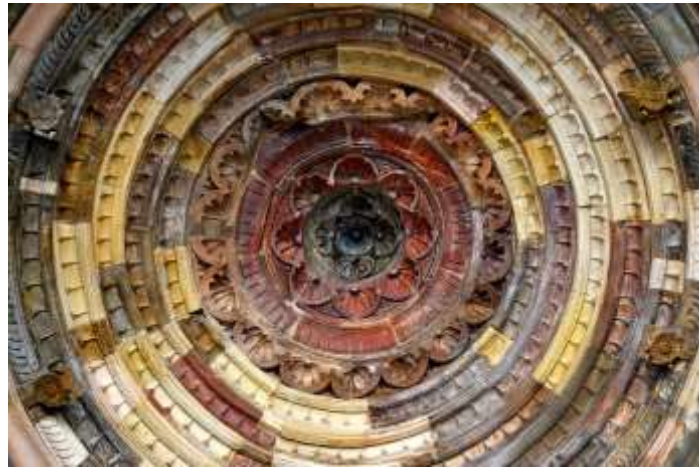
Figure 09. Interior of corbelled dome at Quwwatul Islam mosque (Shapedia, 2017) (Source:- https://www.sahapedia.org/domes-of-delhi retrieved on 30/03/2017)
