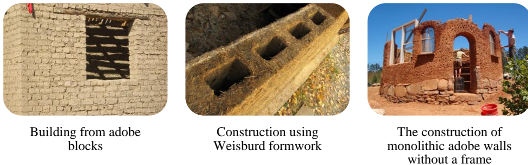
Figure 3. Technologies for the construction of adobe houses
