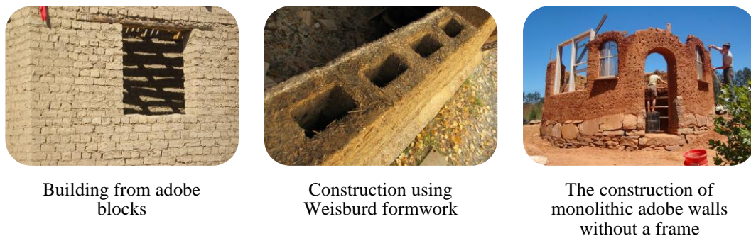
Figure 3. Technologies for the construction of adobe houses
