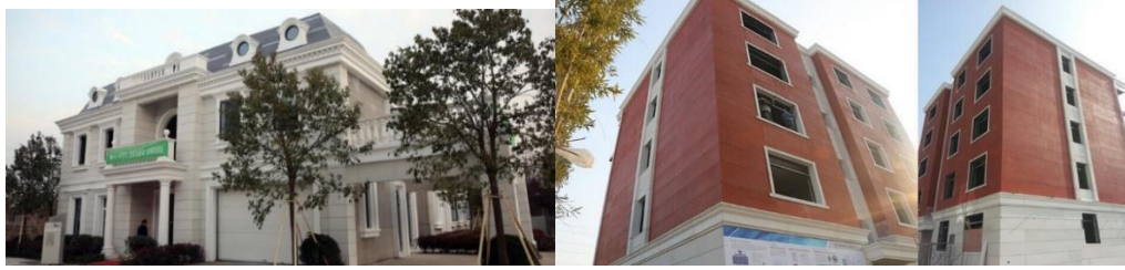
Figure 03. WinSun 3D printed building. WinSun printed Villa (Left) and printed Apartment (Right) Source: AP (2015).
