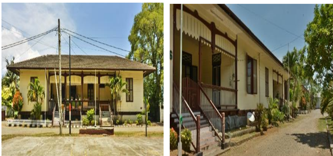
Figure 01. Front facade of the Dutch Dwelling with spacious lot
