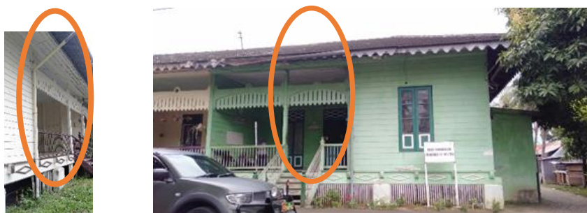
Figure 07. Rainwater gut around the fascia of verandah overhang
