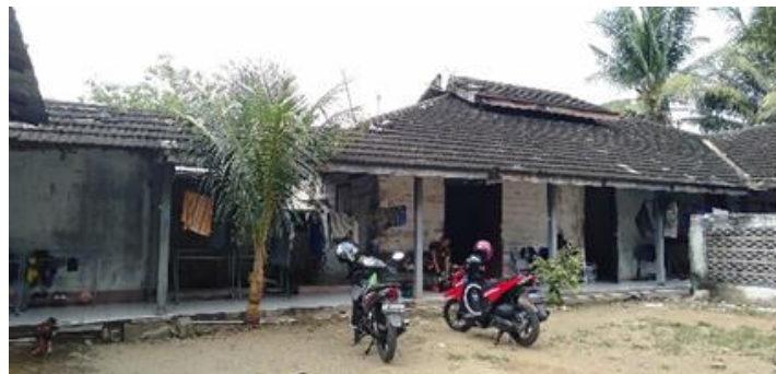
Figure 09. Kitchen roof and façade
