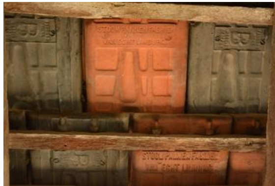
Figure 10. The clay tile roof installed in the Dutch dwelling roof
