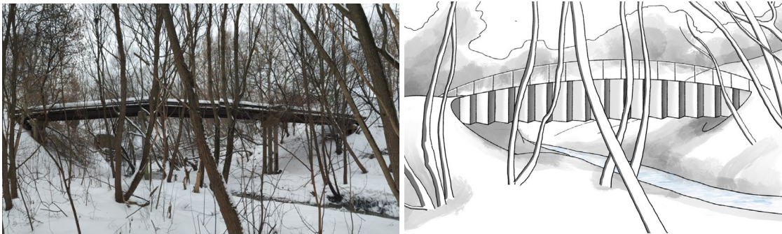
Figure 14. Bridge on the basis of pillars of water supply communications (UN 19). Above - before reconstruction, below - after (drawing by the authors)
