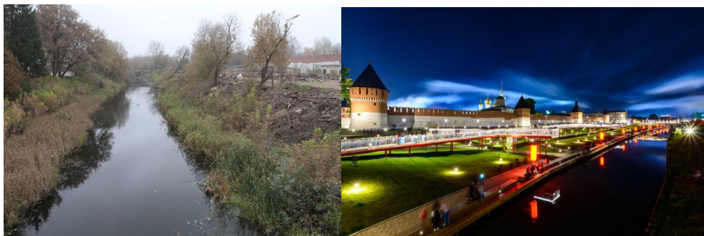
Figure 3. Kazanskaya embankment in Tula: before and after biorevitalization
